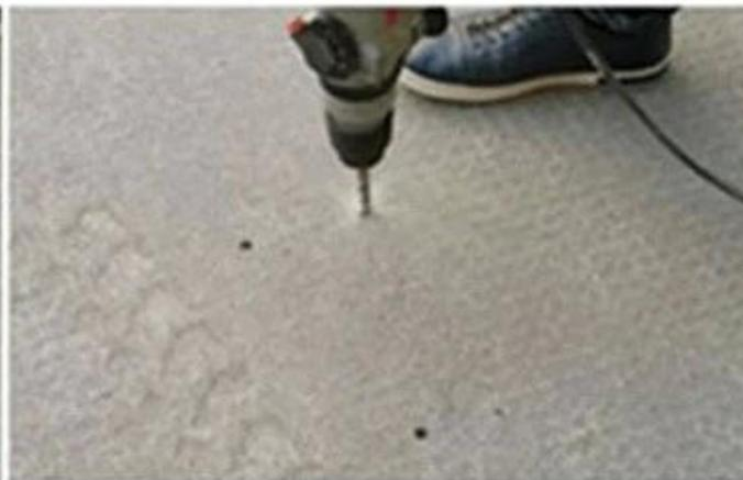
2. Drill a hole for controllable screw installation at the mark.
