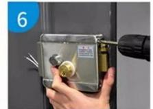
6 Install the front cover plate and secure it with screws. Also, secure the small shell with screws and complete the installation
