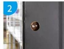
2 Drill circular holes (26.5mm-49mm) according to the size of the lock head outdoors
