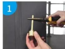
1 Cut the lock cylinder to a suitable length according to the thickness of the door (suitable for door thickness of 30mm-55mm)
