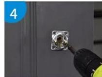
4 Install a three eye board and bamboo screw at the corresponding position indoors
