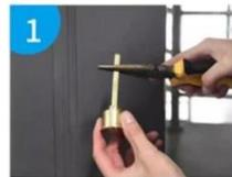
1 Cut the lock cylinder to a suitable length according to the thickness of the door (suitable for door thickness of 30mm-55mm)
