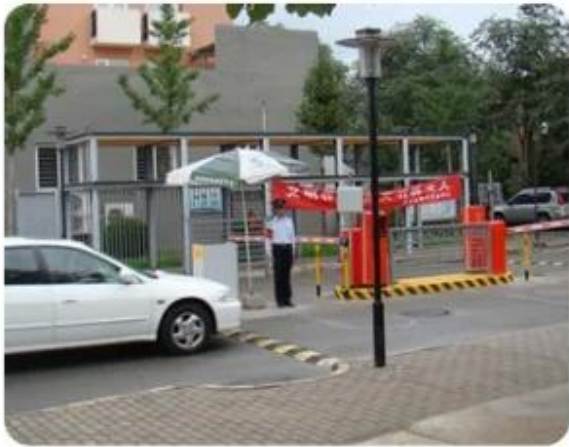
Parking lot vehicle access control system
