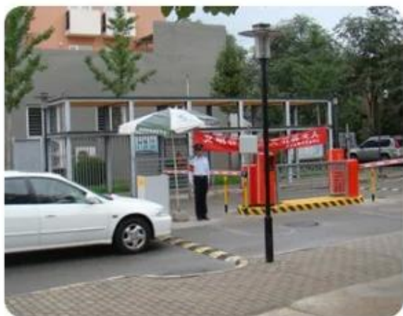
Parking lot vehicle access control system
