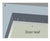
Drill holes based on the marked positions.
