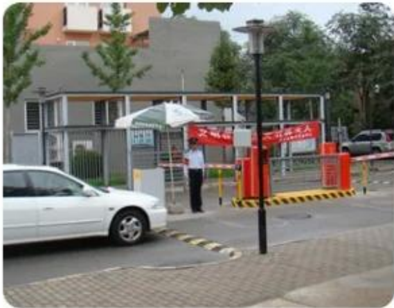
Parking lot vehicle access control system
