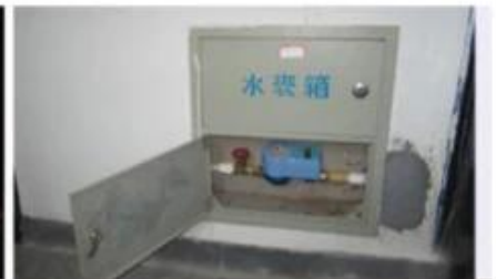
WATER METER BOX
