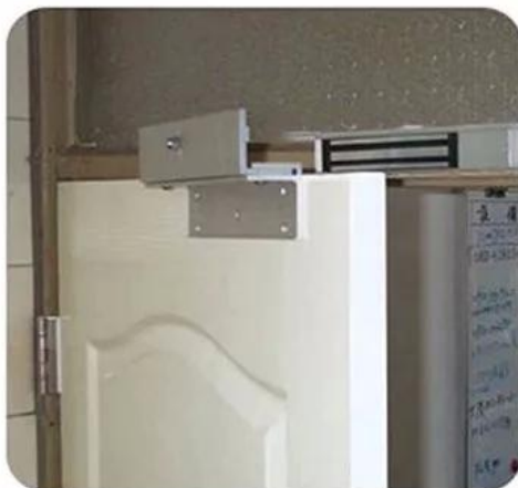
Installation real effect figure
