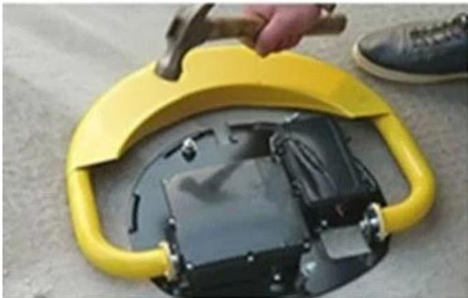
3. Use a hammer to hammer the screw into the drilled hole.
