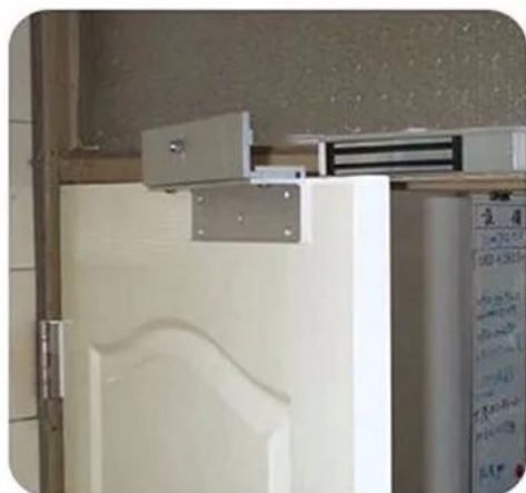
Installation real effect figure
