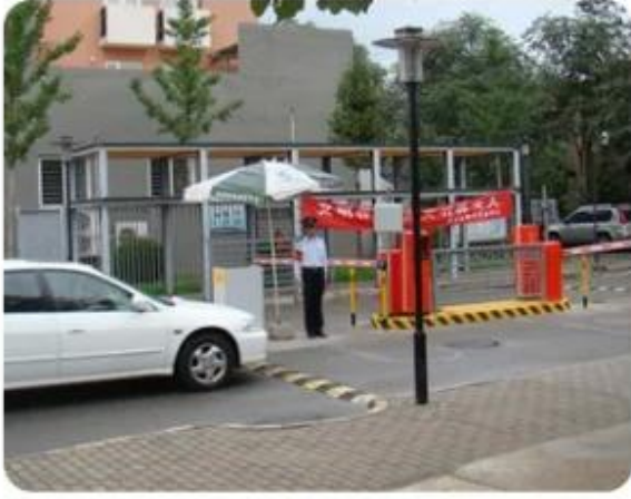
Parking lot vehicle access control system
